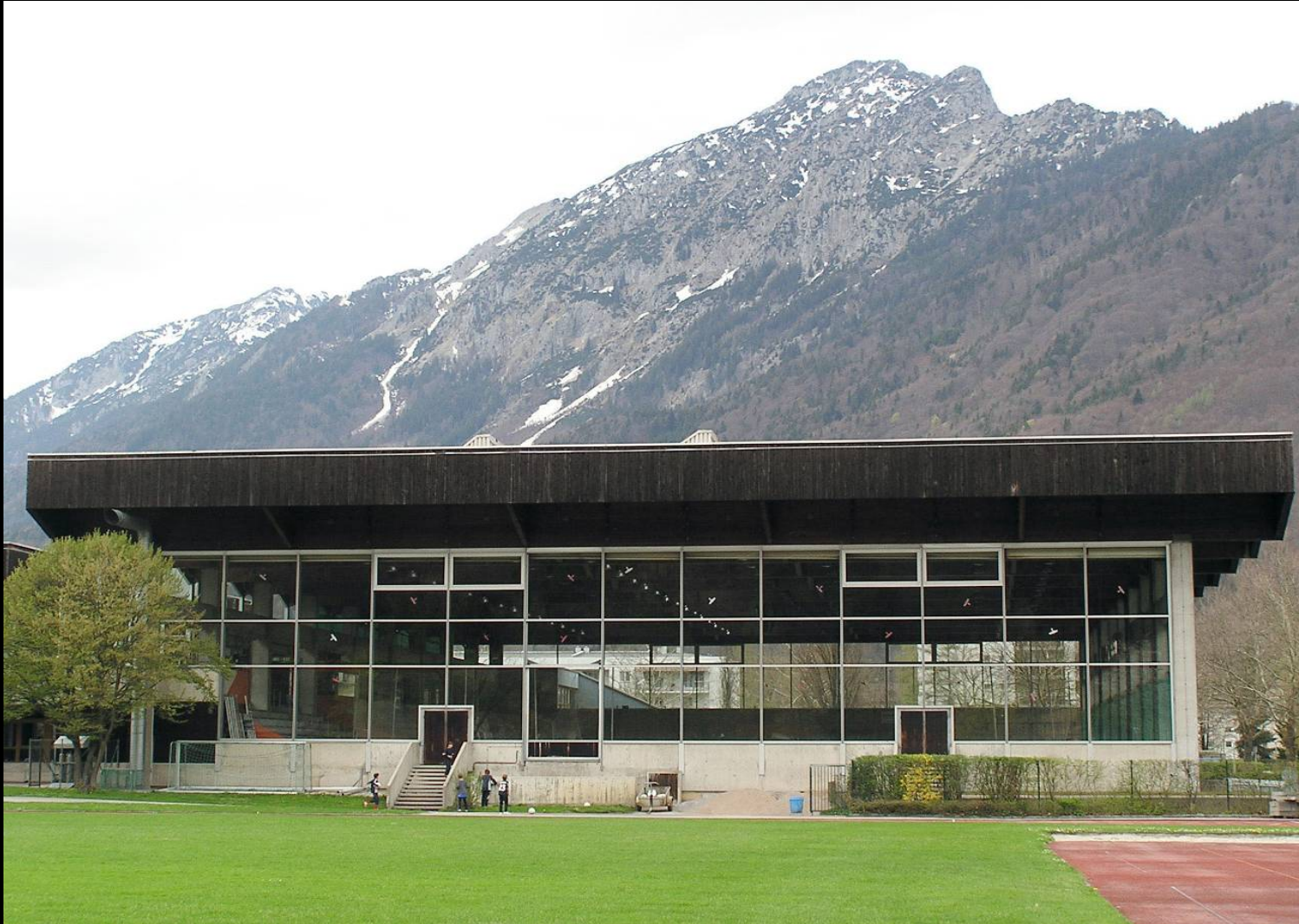
Eishalle Bad Reichenhall – Year of Construction 1971/72
