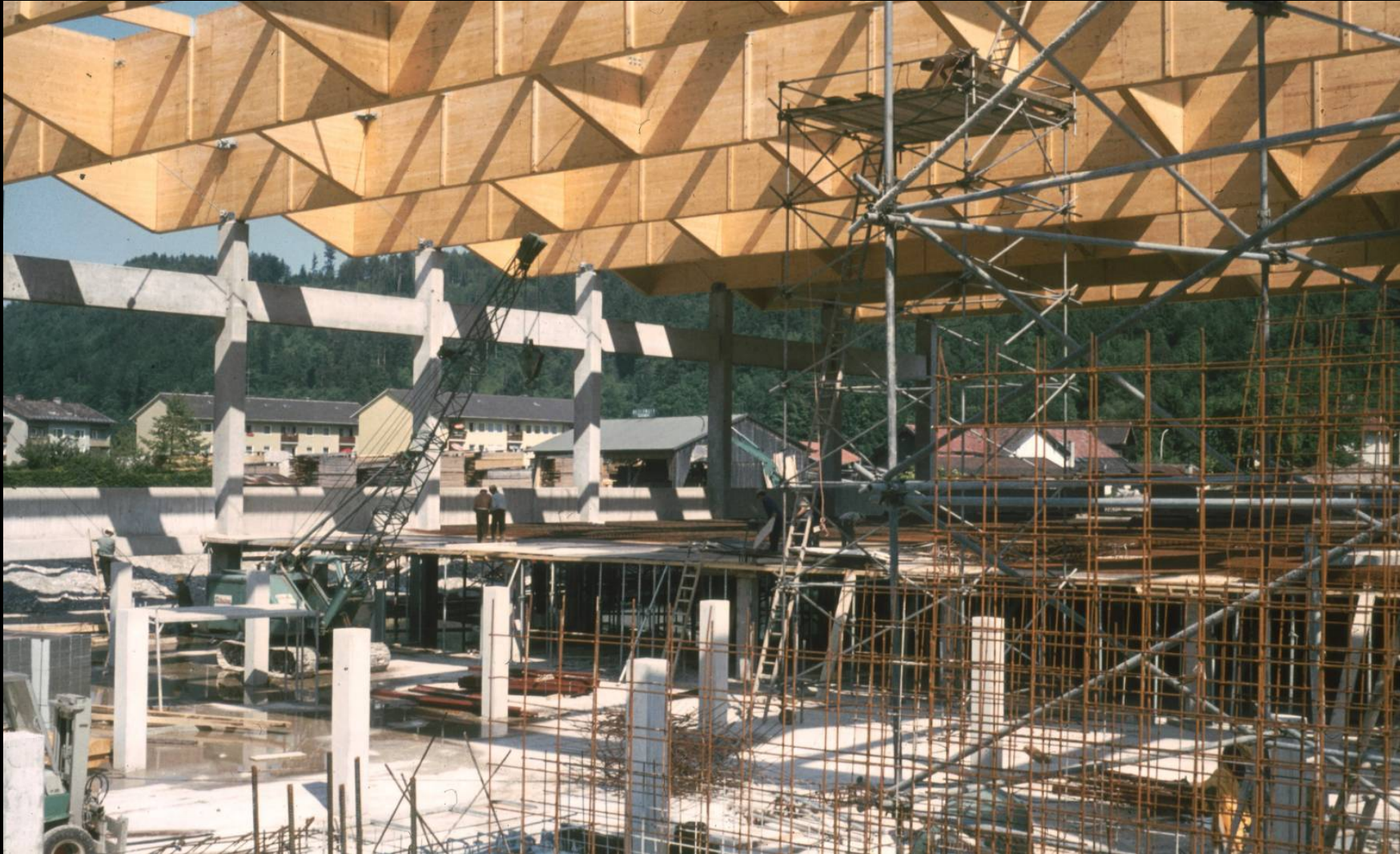
Eishalle Bad Reichenhall – Year of Construction 1971/72
